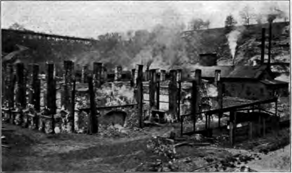
Photograph by F. M. Fultz. KILNS OF THE GRANITE BRICK CO., BURLINGTON, IA. All rights reserved.
